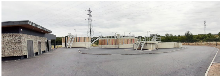
Station de Saint-Ouen-de-Thouberville
